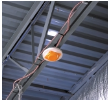
MC cable was selected for this complex project because it was flexible and easy to install.
