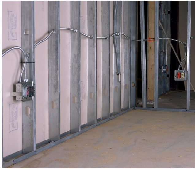
Uni-Fab pre-fabricated branch circuit assemblies save on labor and installation time.
