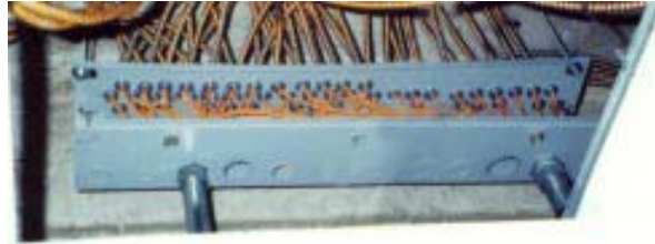
MOF cable is pre-assembled and pre-tested at the factory to save installers time in the field.
