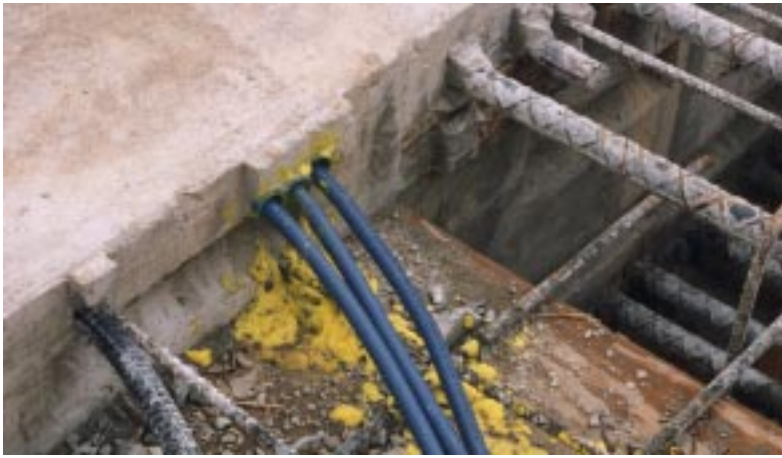
Submerging the cable in concrete or burying it underground is one of the properties of Jacketed MC Cable that makes it unique.
