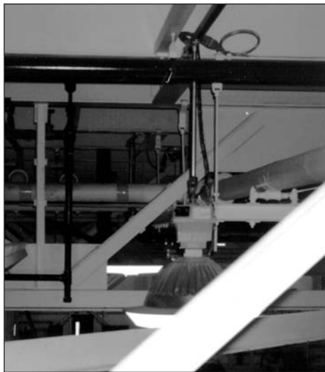
The modularity of Flex3+ allows lighting fixtures to be disconnected and moved without interrupting power to other fixtures down the line.
