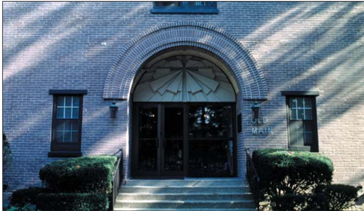
A new voice and data network at Kline Hall of Science, presented a unique challenge for Messiah College, Grantham, PA.
